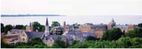
Skyline prior to deconstruction of Motherhouse and St. Mary’s Academy, 2017
